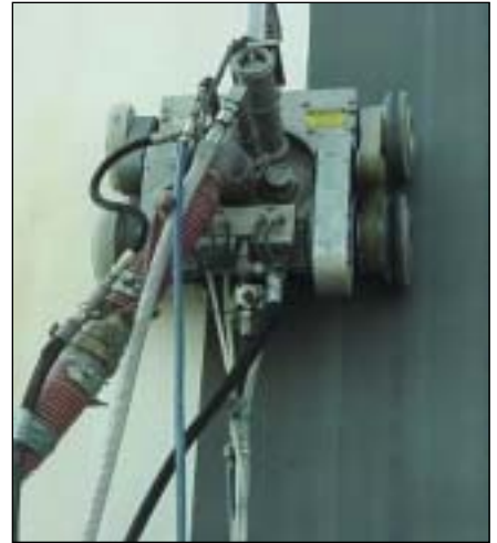
Fig. 2: Absence of water from the crawler as it worked vertically Figs. 2-4 courtesy of NLB Corporation
