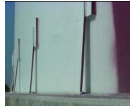
Fig. 4: Bottom straps of tanks primed (left) and topcoated (right)
