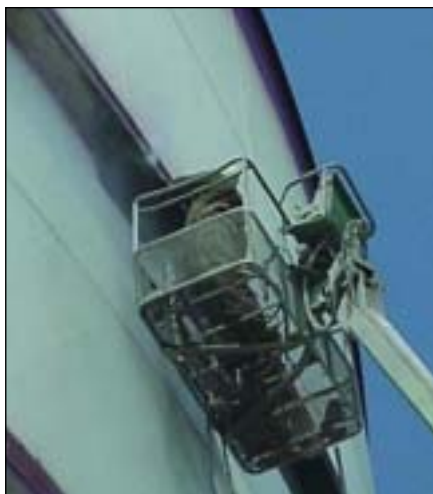
Fig. 3: Manual blasting was used 2 feet above and below the band.
