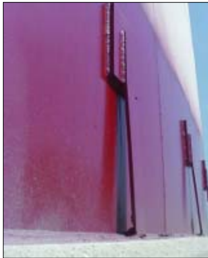
Fig. 4: Bottom straps of tanks primed (left) and topcoated (right)
